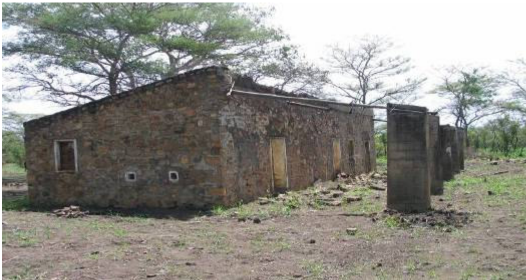
Figure 7 Mission Building before
